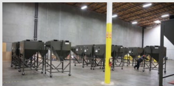
The Philz Coffee roasting facility nears the end of its buildout.
